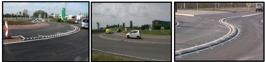
Fig. 21. Lane separation in the turboroundabout [11].
