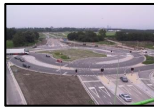
Figure 19. Lane separation in turboroundabout through safety islands [11].
