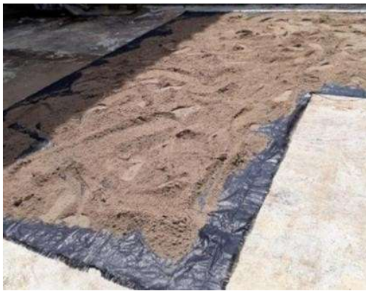
Figure 2. Sand Preparation Process
